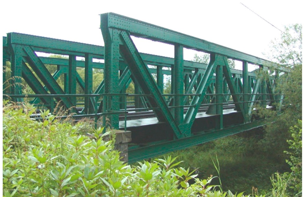
Figure 7. View of the bridge in Turany.
