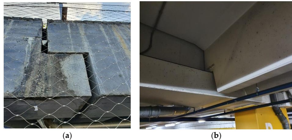
Figure 1. General view of a dapped-end beam connection: (a) rectangular dapped-end beam; (b) double-T dapped-end beam.
