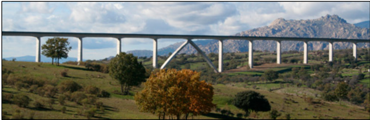
Figure 2. Viaduct “Arroyo del Valle” (E-2 structure) (Adif-AV, Mitma).
