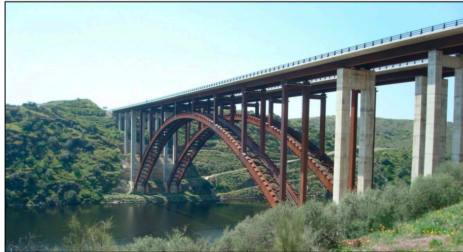
Figure 1. Viaduct “Arcos de Alconétar” (E-1 structure) (Mitma).
