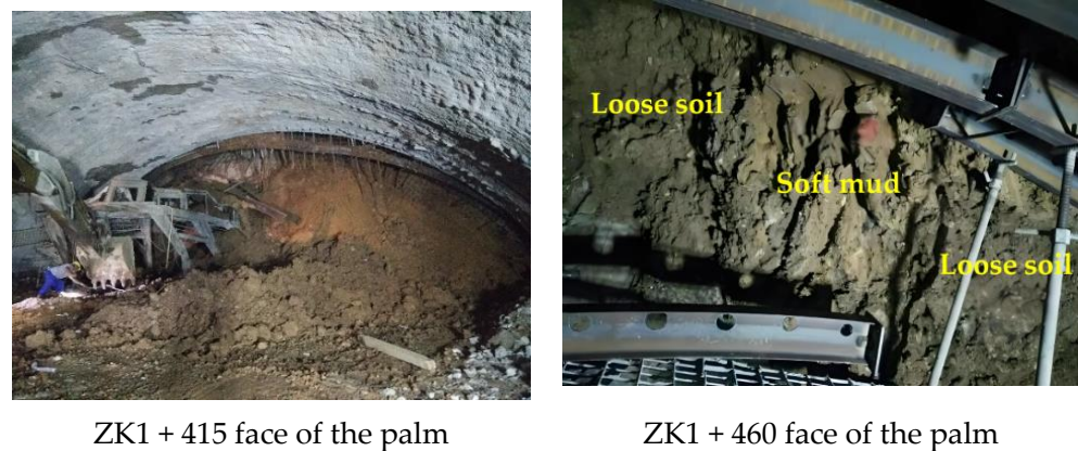
Figure 7. Typical surrounding rock of tunnel face.
