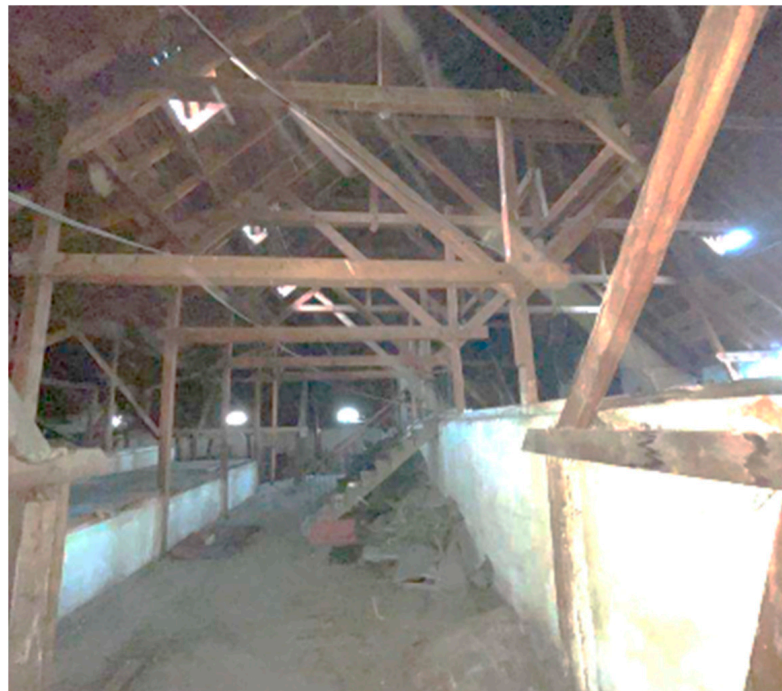
Figure 5. Image displaying the uninsulated attic.
