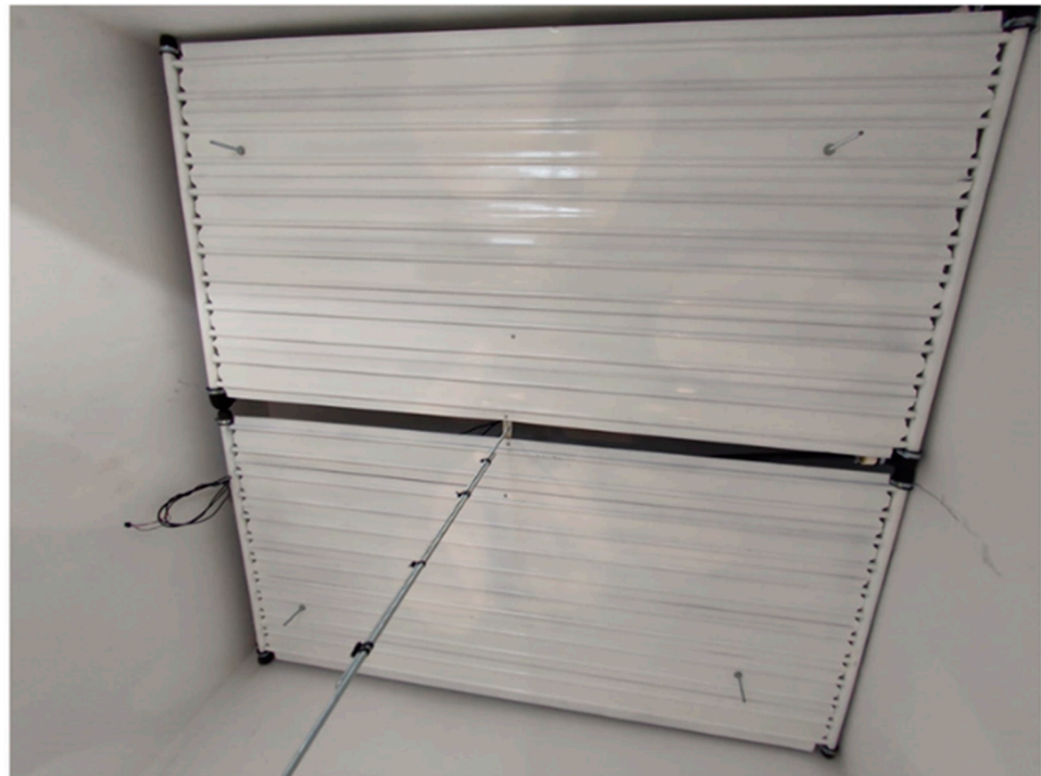
Figure 4. The placement of the collector panels.
