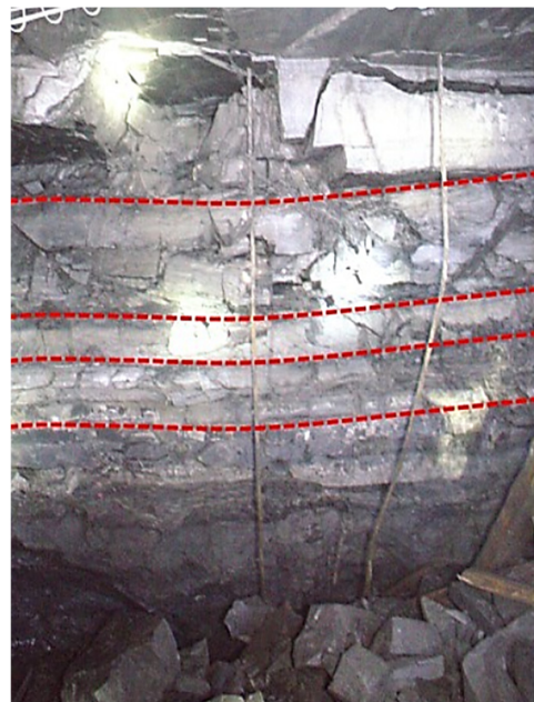
Figure 3. Composite Roof of Roadway Exposed On Site.
