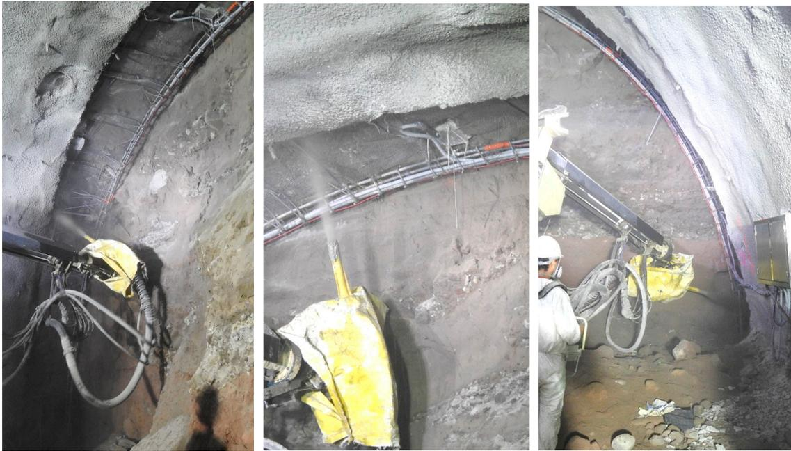
**Figure 11.** Placement of the first layer of shotcrete with 10 cm thick fibers, covering the periphery of the tunnel vault and the instrumented radial pressure cells. Photographs taken by the author, 2021.
