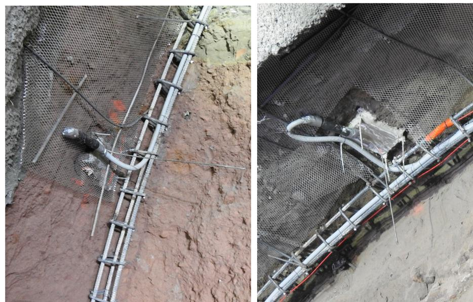
**Figure 10.** Finally, the pressure transducers are protected with steel ducts and are channeled to the Datalogger where they are connected. Photographs taken by the author, 2021.
