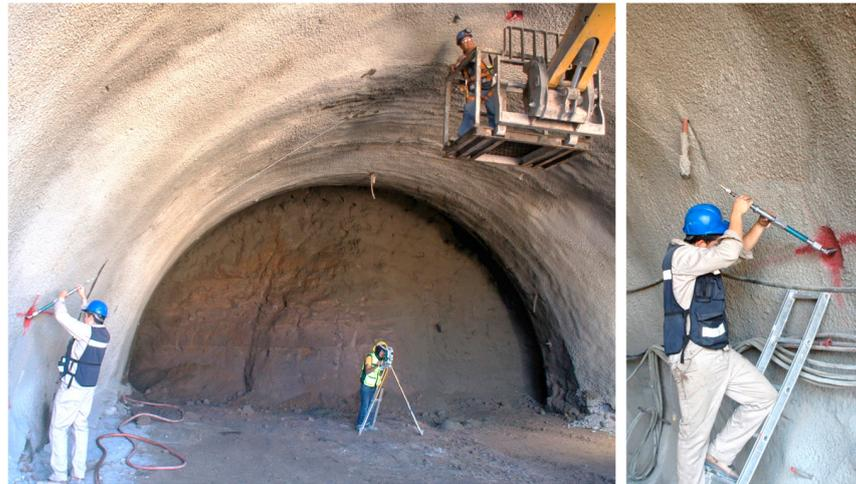
**Figure 8.** Measurement of convergences during the excavation of the upper half section. Photographs taken by the author, 2021.
