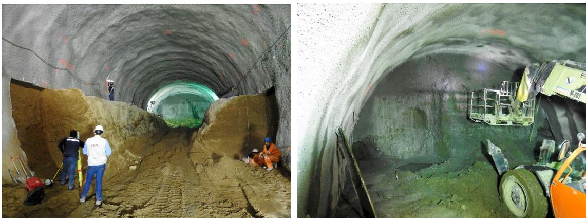
Figure 5. Excavation of the complete upper half section with a central core. It shows the poor quality of the soil and the presence of water seepage.
