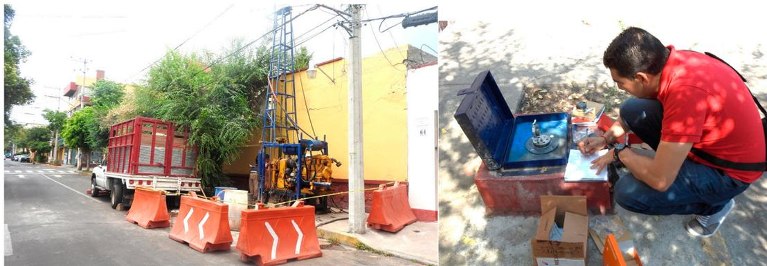
**Figure 7.** Drilling for the installation of the extensometer and measurement of the instrument. Photographs taken by the author, 2021.
