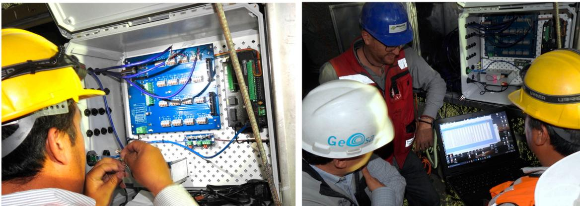
**Figure 12.** Photograph showing the connection of the instruments to the Datalogger. Once connected, the first readings are taken on a laptop using the Logger Net software version 4.5.
