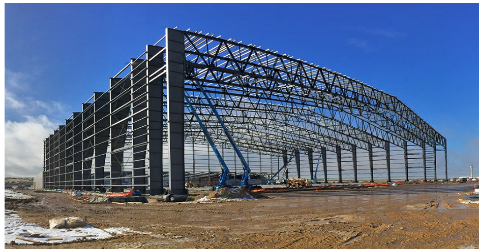
Figure 1. Steel building constructed using cold-formed steel channel sections.
