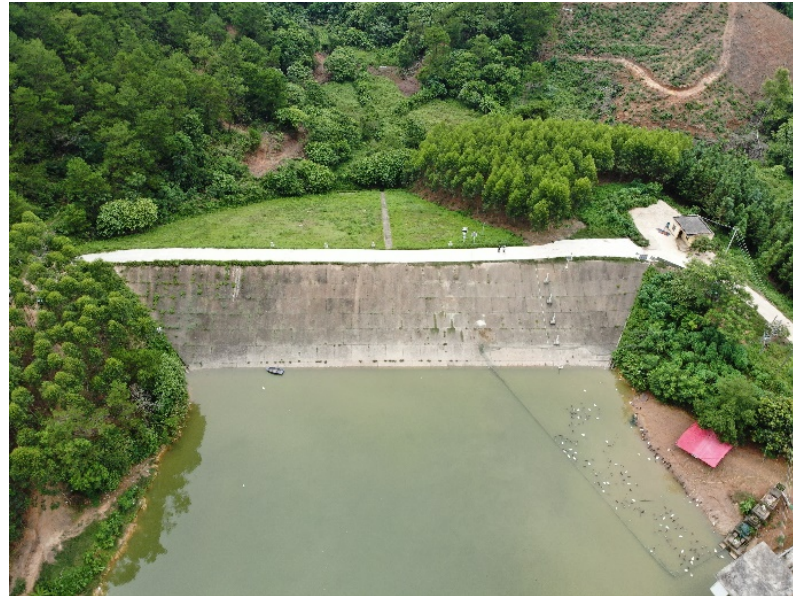
Figure 21. Photograph of the small reservoir dam for Case 2.
