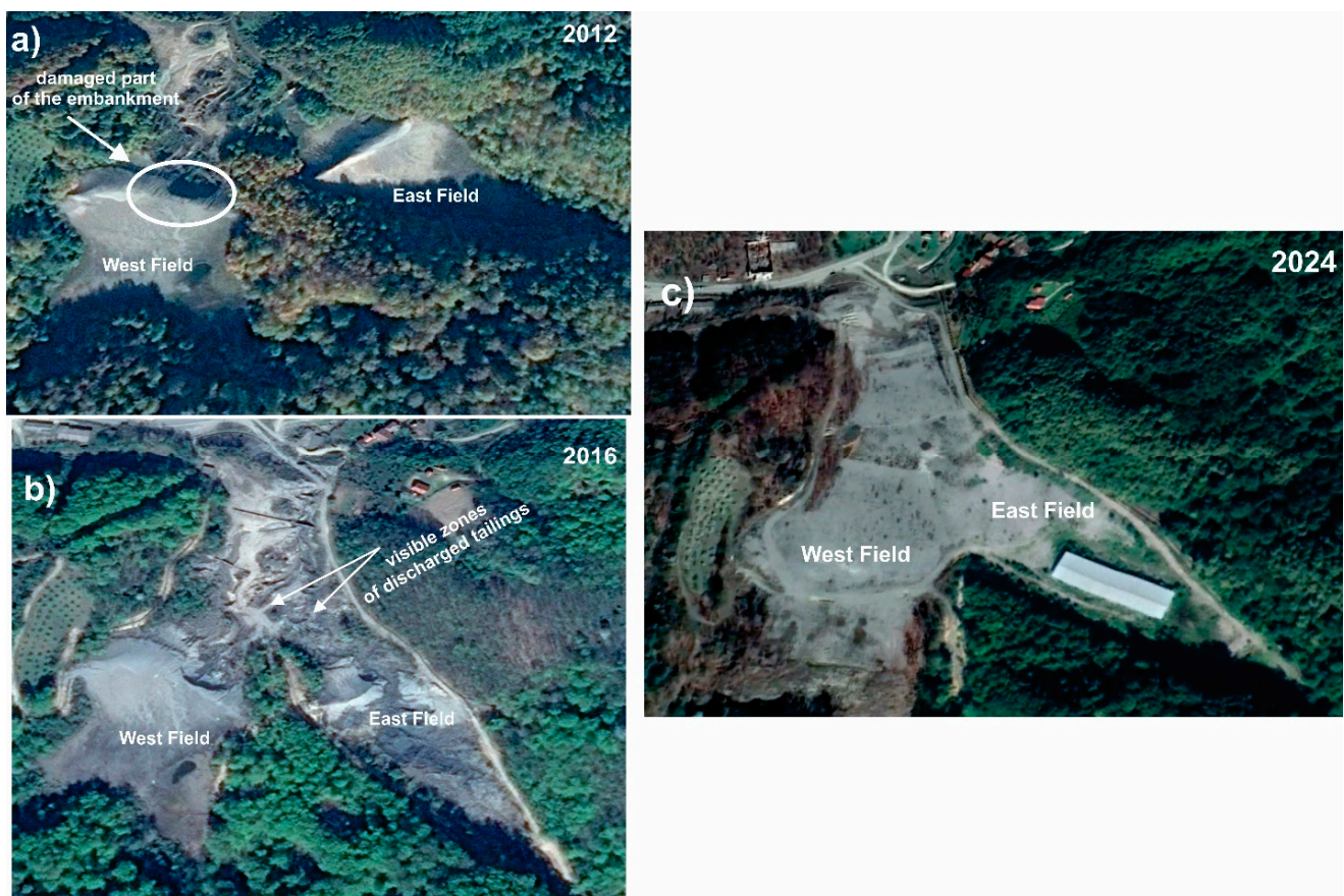
Figure 3. The flotation TSF of the mine “Stolice”: (a) image from 2012, before the accident; (b) image from 2016, after the accident and before rehabilitation; (c) image from 2024, after rehabilitation [17].
