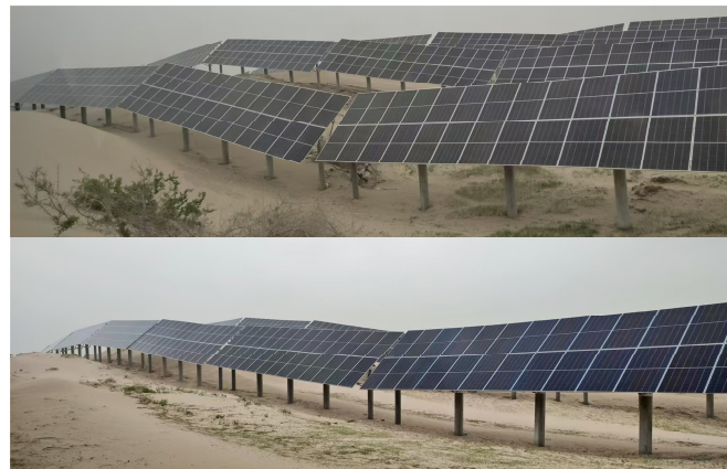
Figure 2. The actual inspection of desert PV power plants.
