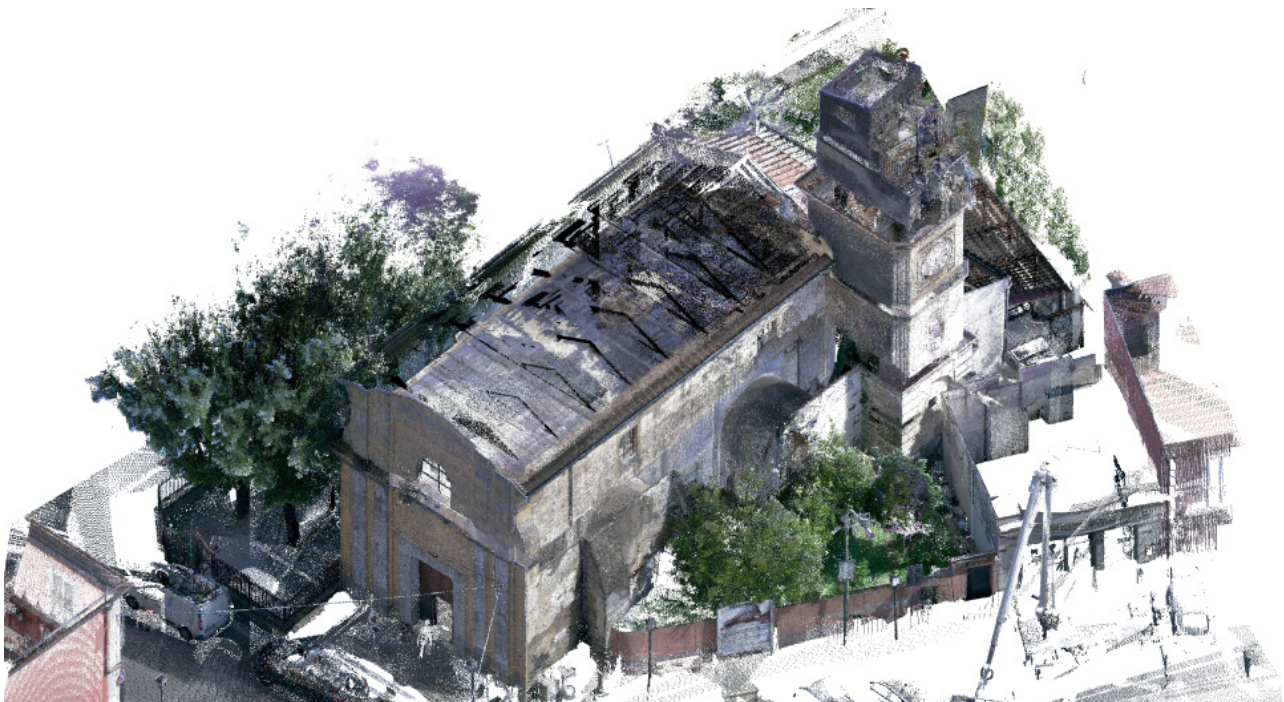
Figure 2. Global view of the 3D laser scanner survey.
