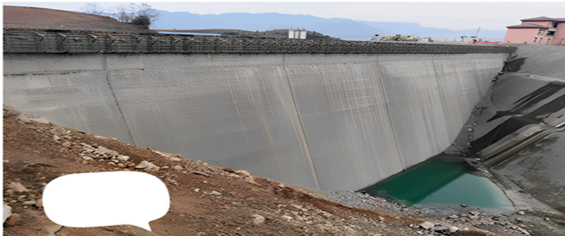
Figure A1. During the construction of Lengshuihe Auxiliary CSGRD.
