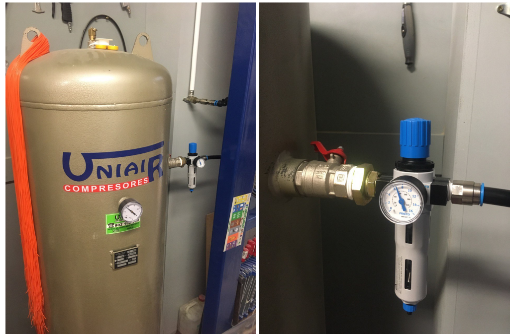
Figure 3. Air tank (left) and details of its outflow pressure regulation control (right).
