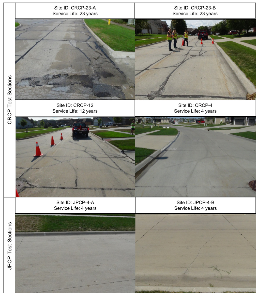
Figure 6. Typical pavement conditions of the six test sites.
