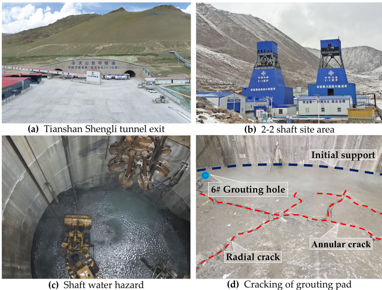
Figure 15. Overview of the shaft's engineering.
