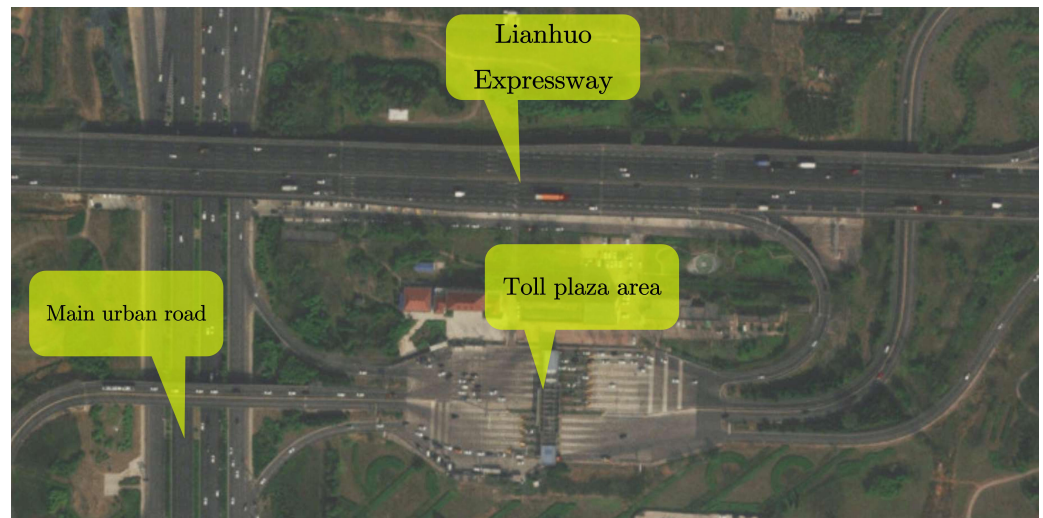
Figure 2. The Liulin toll station and its surrounding roads.
