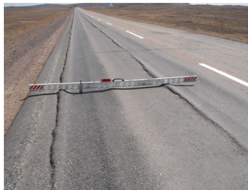
Figure 15. Plastic strains (the depth of the rut is more than 60 mm) in asphalt concrete layers of the highway “Ekaterinburg-Almaty” (km 1903.1—Karaganda Region, Kazakhstan).
