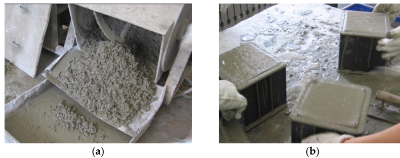
Figure 2. Photographs for GB concrete mixing and casting: (a) anchor type of concrete mixer; (b) elimination of entrapped air from specimens using vibration table.
