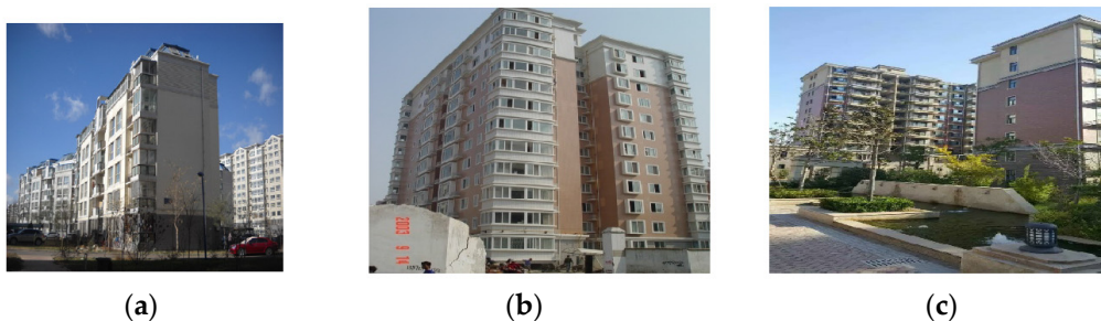
Figure 2. Residence pilot projects using CMR wall panel structure with energy-efficient blocks. (a) Xing-Guang Hua District in Yin Chuan, the Ningxia Hui Autonomous Region; (b) Geng-xin-street District in Xi'an, Shanxi Province; (c) Zhong-zhou-yu-fu project, in Lankao, Henan Province.
