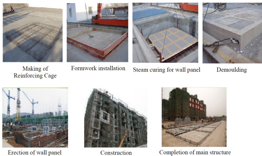
Figure 4. Production and assembly of CMR wall panel structure with energy-efficient blocks.
