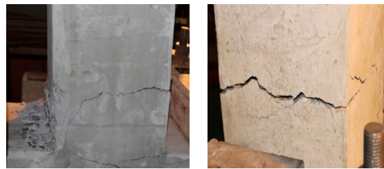
Figure 8. Crack and failure mode of column 6#.
