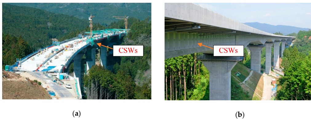
Figure 1. Shintogawa Bridge in Japan (completed in 2013): (a) Top view; (b) Side view. CSWs: corrugated steel webs. CSWs: corrugated steel webs.
