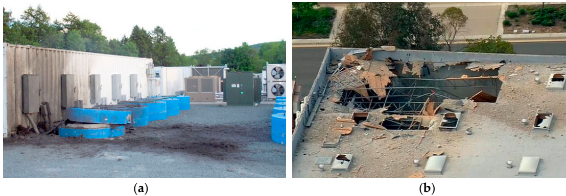
Figure 2. (a) Impressions of the accidents at Beacon Power in Stephentown [8]; (b) Quantum Technologies flywheel-plant in San Diego, USA [9].
