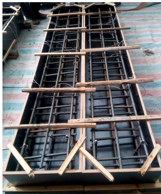
Figure 4. Reinforcement layout in frame work before casting.
