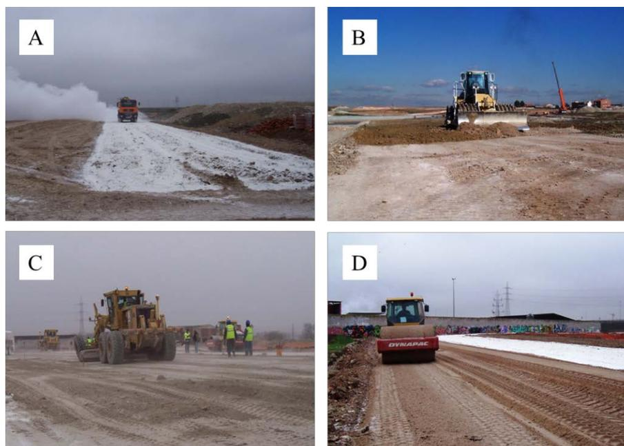
**Figure 7.** Embankment execution procedure. (A) Extender line on the dry soil; (B) mixed with lime and clays; (C) profiling motor grading layer; (D) compacting process.
