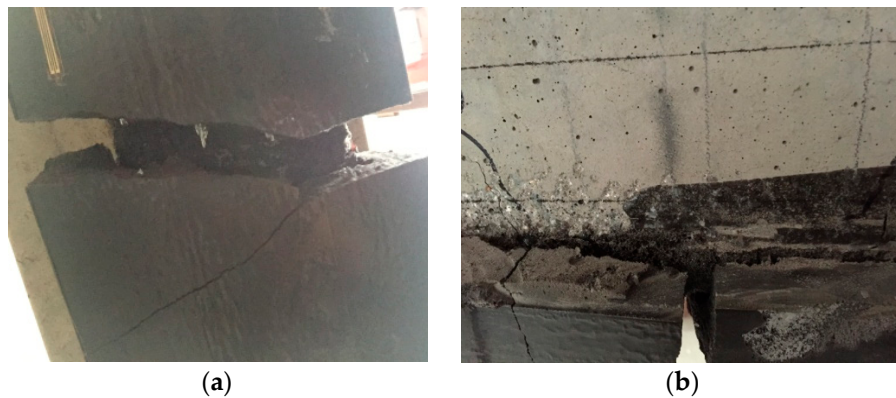
Figure 6. Flexural failure. (a) Bottom transverse fracture; (b) CNFPUC is separated from the concrete.
