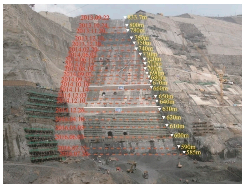
Figure 6. Detailed excavation schedule of the rock slope.
