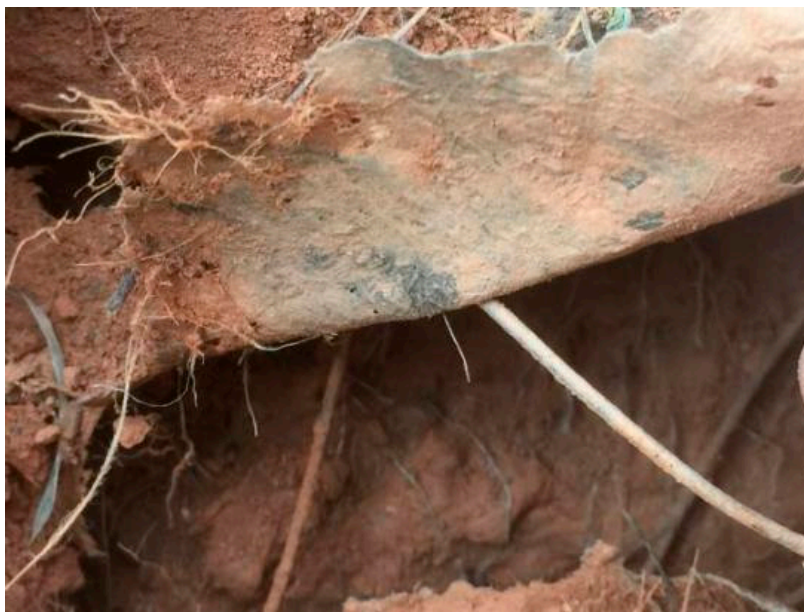
Figure 14. Penetration of the plant root system into the curing agent layer.
