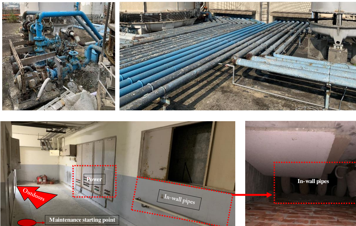
Figure 4. Photographs of outdoor (top) and indoor (bottom) layout to which BARMS was applied.
