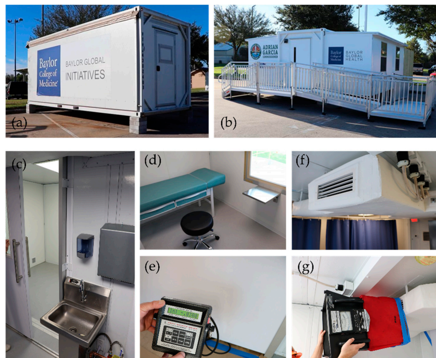
Figure 2. Photographs of the COVID-19 Smart Pod isolation clinic. (a) Folded unit in its transport mode; (b) Expanded container-based clinic with an ADA-compliant ramp; (c) Entrance to the isolation room; (d) Interior in the isolation room features bleachable surfaces; (e) A micromanometer shows measurements of negative pressure in the isolation room; (f) One of the air supply outlets of the air distribution system; (g) Positive pressure evaluation in one of the air supply outlets using a velometer.
