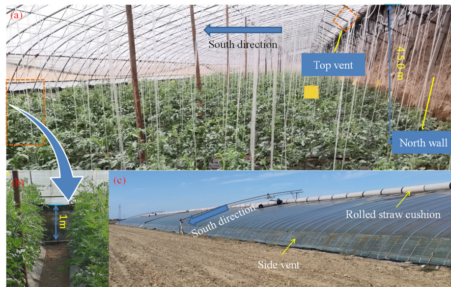
Figure 1. Photos of the sunken solar greenhouse. (a) Inside view during tomato planting. (b) A view of the sunken soil inside. (c) Outside view in winter. The front plastic cover faces south, and the rolled straw cushion is on the top of the roof.
