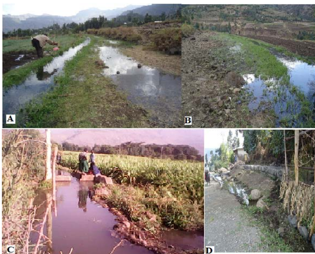
Figure 6. Water seepage in the Woyeneyie (A) and Gedober scheme (B); Seepage loss in the traditionally built irrigation canal constructed by beneficiary farmers themselves in Sanka (C); and overtopping on the main canal in Sanka's traditional irrigation system (D), respectively.
