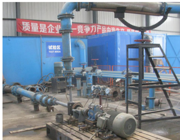
Figure 3. Hydraulic performance test bench.
