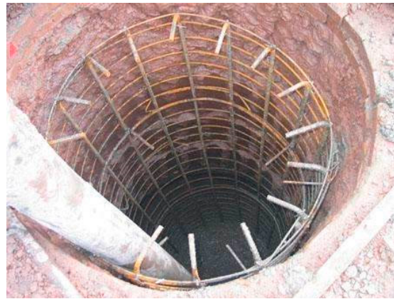
Figure 1. The rough surface of sidewall.
