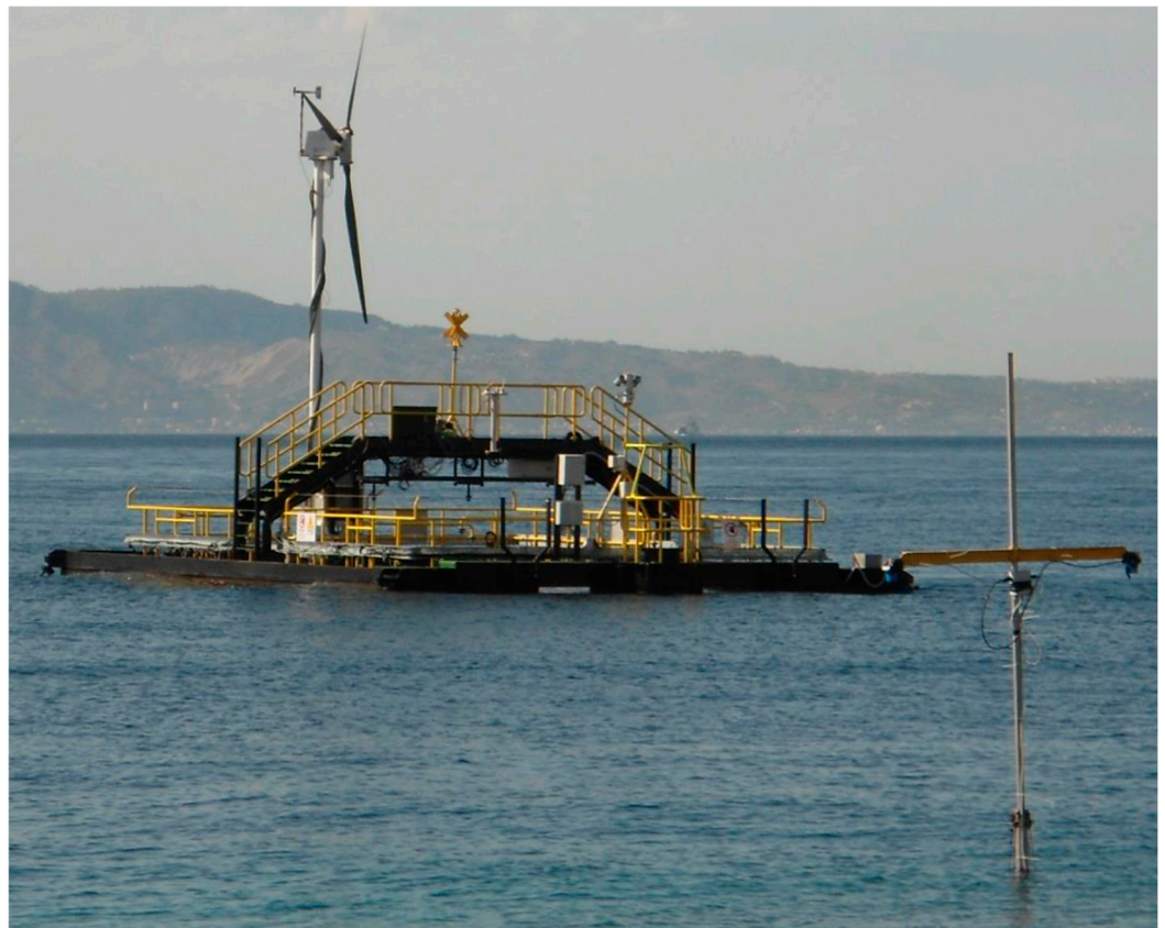
Figure 1. Photo of BGF platform installed at NOEL.
