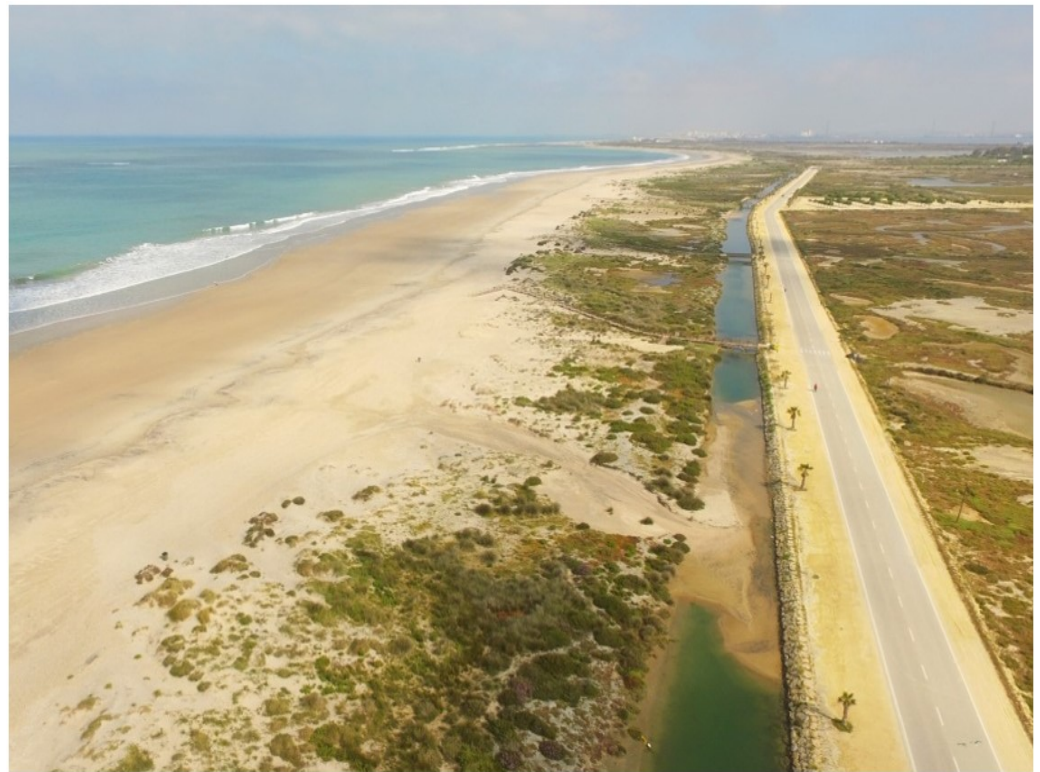
Figure 11. Aerial picture of Camposoto Beach presenting a washover fan located in Section 1. Source: Talavera [34].
