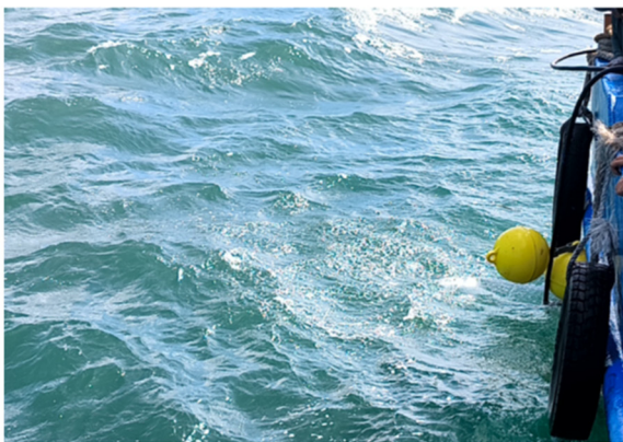
Step3: Deploy cement heavy block, lay cable and floats down
