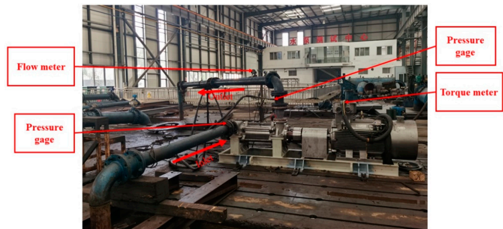
Figure 5. Test system of multiphase pump.
