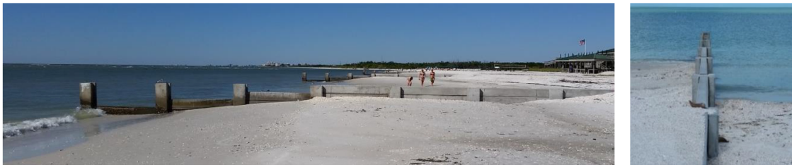
Figure 2. Photos of the king-pile groins on Big Hickory Island, FL.
