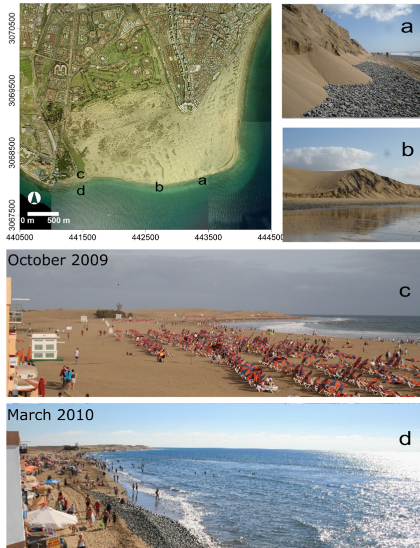
Figure 2. Beach and dunes erosion due to high-energy storm waves of Winter 2009/10. (a), dune avalanching (b), eroded dune front (c) Pre-storm beach (October 2009) and (d) Post-storm beach showing shoreline retreat after 17th February 2010.
