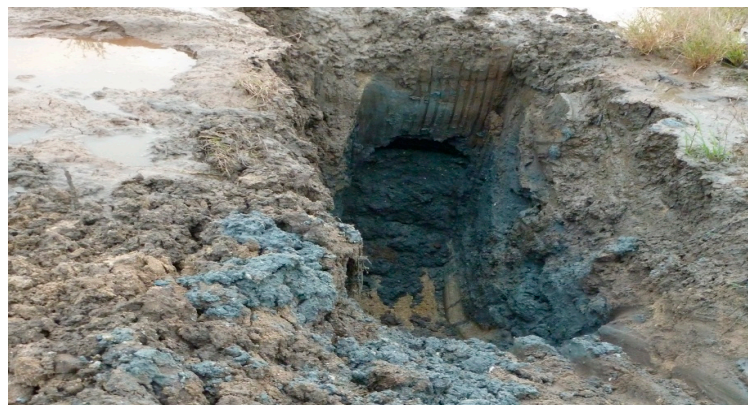
Figure 7. Site excavation of marine soft soil.
