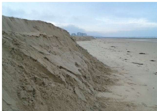
Figure 13. Ground photograph of the berm following the high water of 12 November.
