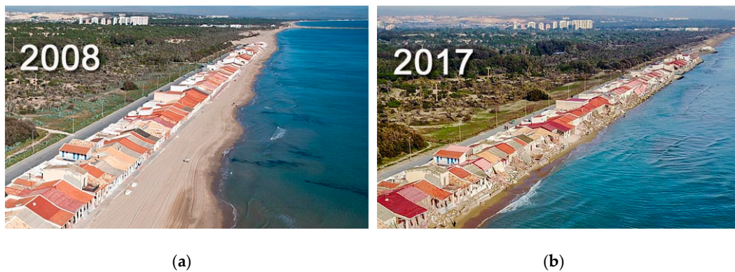
Figure 1. Effects of the shoreline recession on nearby buildings, caused by anthropogenic stress: (a) shoreline in 2008; (b) same view in 2017.
