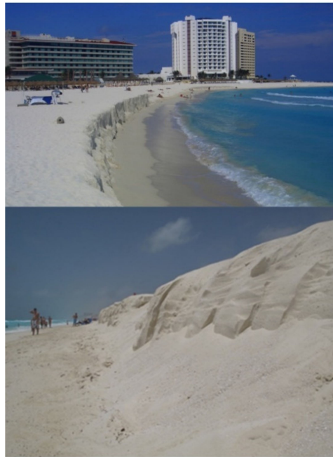
Figure 12. The second beach nourishment was carried out in June 2010. By October 2010 the beach had developed a scarp of almost 2 m height as seen in both photographs.
