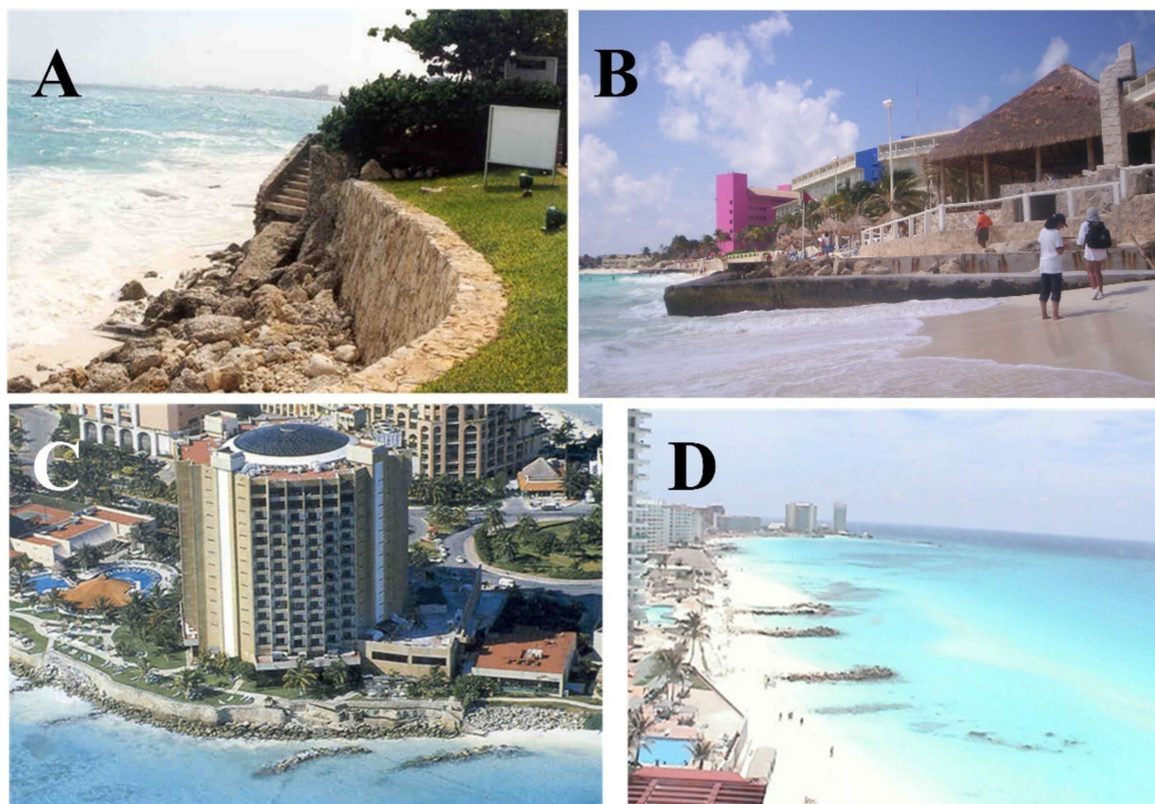
Figure 3. Examples of inadequate solutions implemented 1988–2004. Vertical walls (panels A and B); detached structures (panel C) and groins (panel D).
