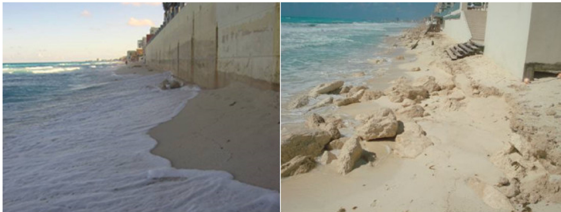
Figure 8. View of the beach at Cancun in 2009, before the second nourishment. Waves attacking the hotel facings (left) and rocks left behind after erosion (right).
