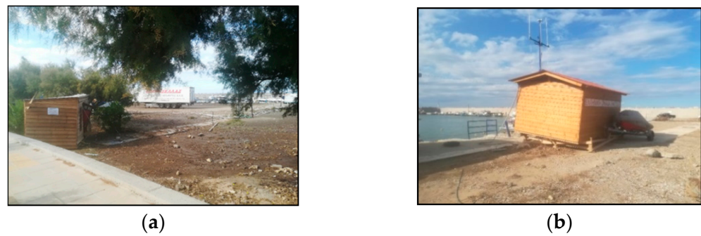
Figure 21. Site K2. In position D (Figure 19), a wooden structure of the cultural association of Karlovasi was dragged away from its initial position for ~10 m (a); in position E (Figure 19), a similar structure was displaced upwards (b) (photos credit, M. Gogou).
