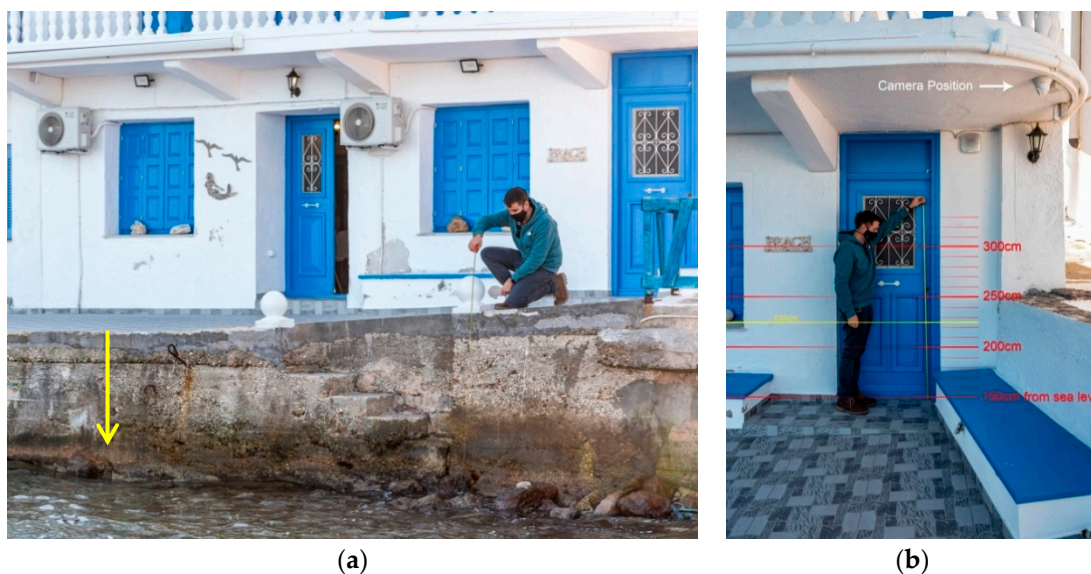
Figure 23. Site K4. Team member performed measurements and found the house entrance level at a height of \sim 1.50 m asl, including the co-seismic uplift of \sim 20 cm (yellow arrow) (a). Heights asl in the door below the security camera (white arrow) are marked (b) (photos credit, M. Thravalos).
