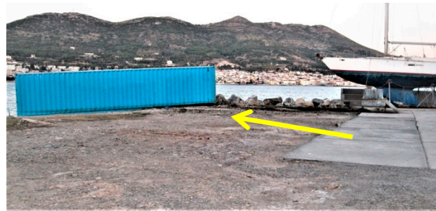
Figure 17. Site V8. The tsunami moved an iron container, from its initial position on the pier, by \sim 8 – 9 m (arrow). In the background, the Vathy town is seen (photo credit, I. Triantafyllou).
