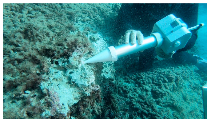
Figure 9. Test of the mortar injection tool (Tech4Sea srl 2020).
