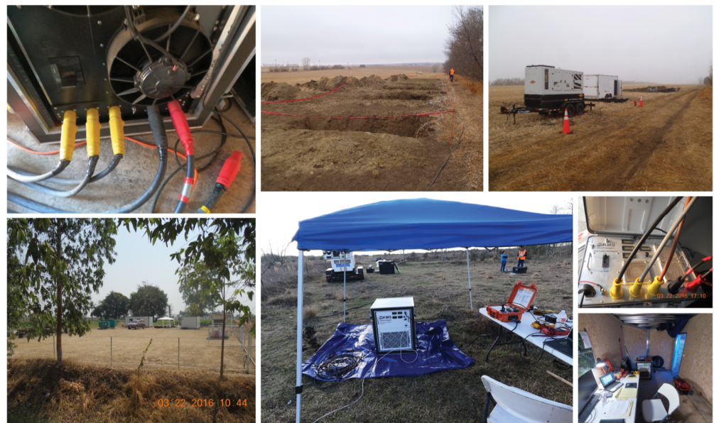
Figure 9. Field images of various components of the transmitter equipment. At the top left is the power connection of the 150 kVA transmitter switch box (back view). Its front view in the field is shown in bottom center. At the top center are pictures of the electrode puts where the current injecting electrode are buried. At the top right is a view of the 150 kVA generator and observer trailer (switch box is inside) used for 24 h continuous for 5 weeks operation partially at minus 20 °C. An inside view of the trailer is at the bottom right. On the left side is a transmitter site set up as camp in the tropic in an oil field.
