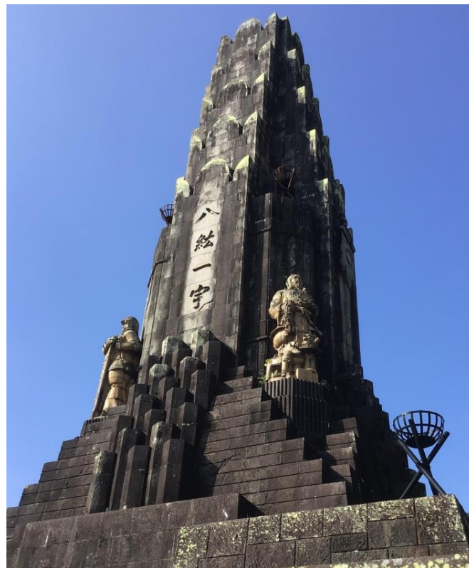
Figure 2. Hakkō Ichiū Tower, Miyazaki, Japan. © Hatena Blog. 2022.
