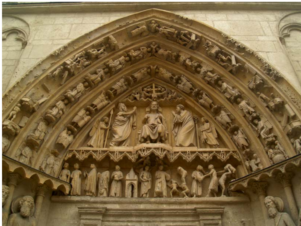
Figure 2. Tympanum of the Coroneria Portico, c. 1245–1257. North façade of the Burgos Cathedral.
